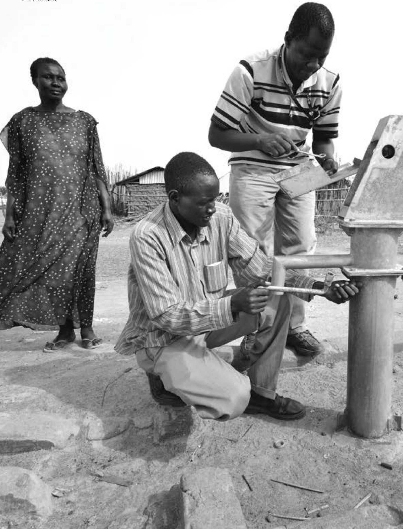
Majdi Abduharaman (right) and Abraham Thom repair the hand pump on a well in Bor, a city in South Sudan's Jonglei State that has been the scene of fierce fighting in recent months between the country's military and anti-government rebels. © ACT/Paul Jeffrey
